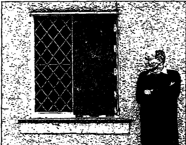
Colin Seymour and the broken window yesterday
